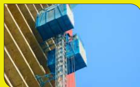
High rising self erecting Rack & Pinion type Hoist
